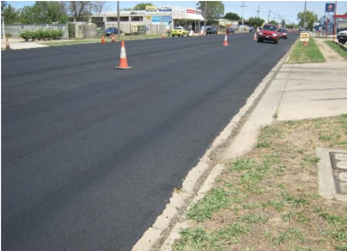
Installing the Micro Surfacing
