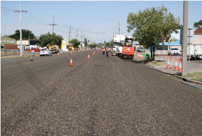
Installing the seal February 2014
