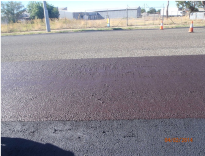
Installing the Micro Surfacing
