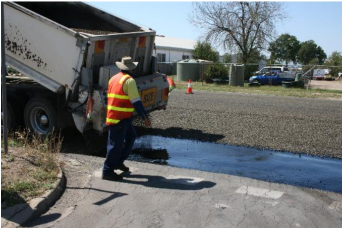
Installing the seal February 2014
