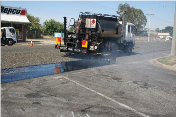
Installing the seal February 2014
