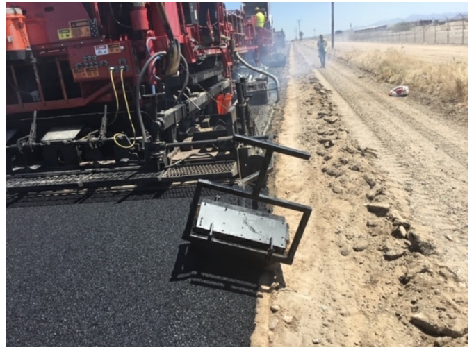
Hot in Place Repaving/safety edge
