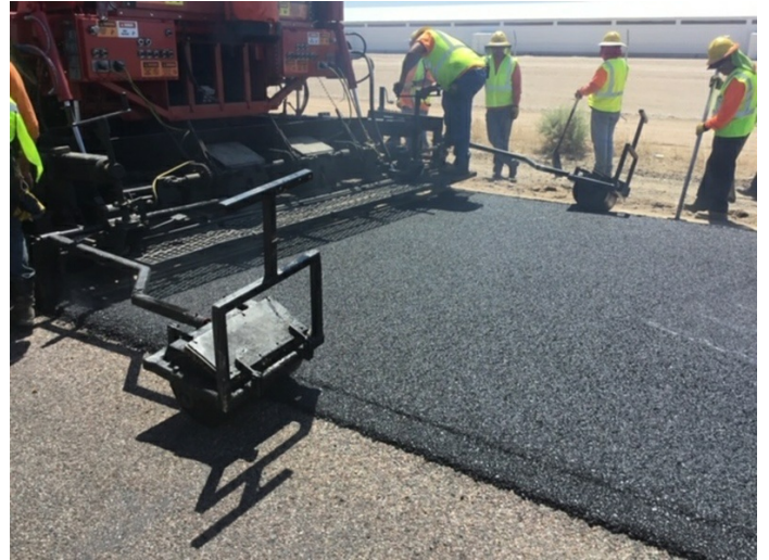
Final 1" recycled layer under 1" new layer AR.
