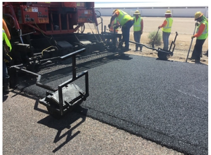
Final 1" recycled layer under 1"new layer AR.
