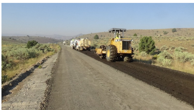
Compaction on Juntura Cutoff
