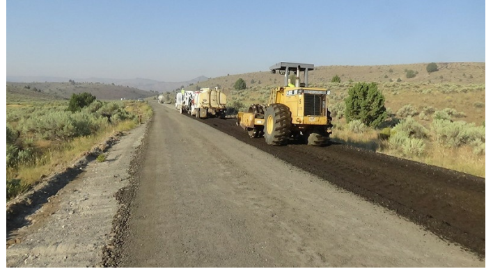
Compaction on Juntura Cutoff
