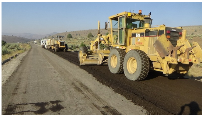
Grading and compaction
