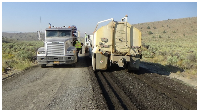
Keeping the road open during construction
